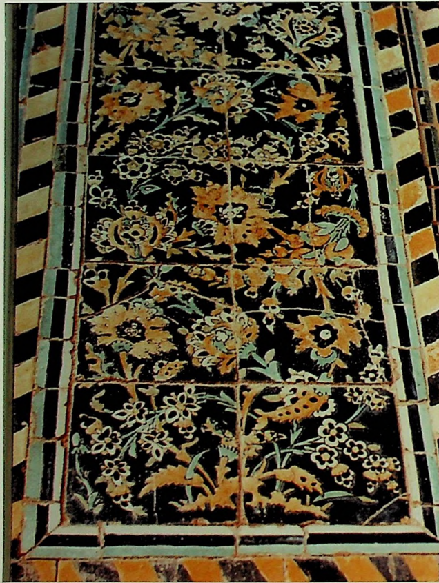
Fig 17: Detail of cuerda seca tile panel in courtyard of Masjid-i Shah, Isfahan: 1611-66. Book 6.
