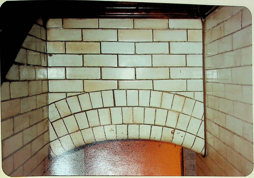
53. Detail of enamelled brickwork
