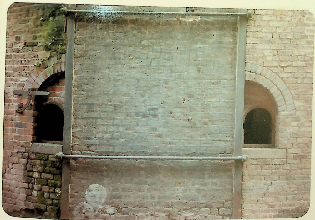
24. Furnace at the base of square chimney.
