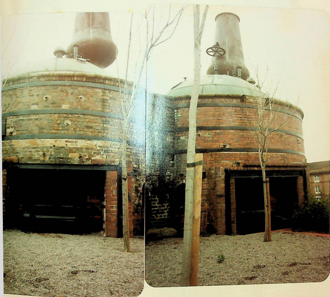
31. The Furnaces under the stills
