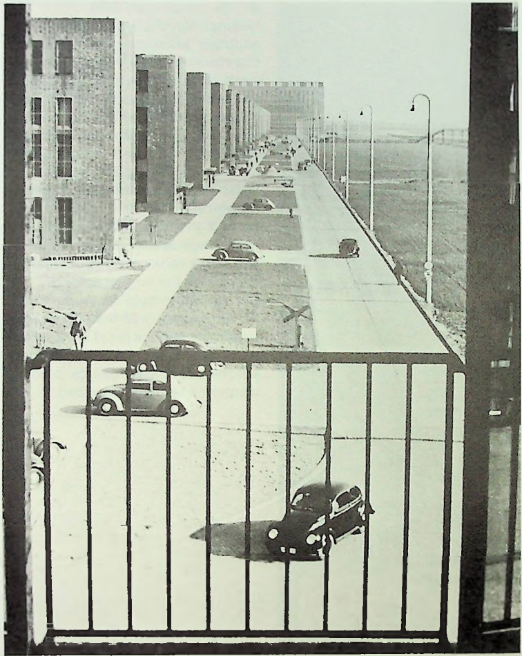
Fig. 19: View along front of factory.
