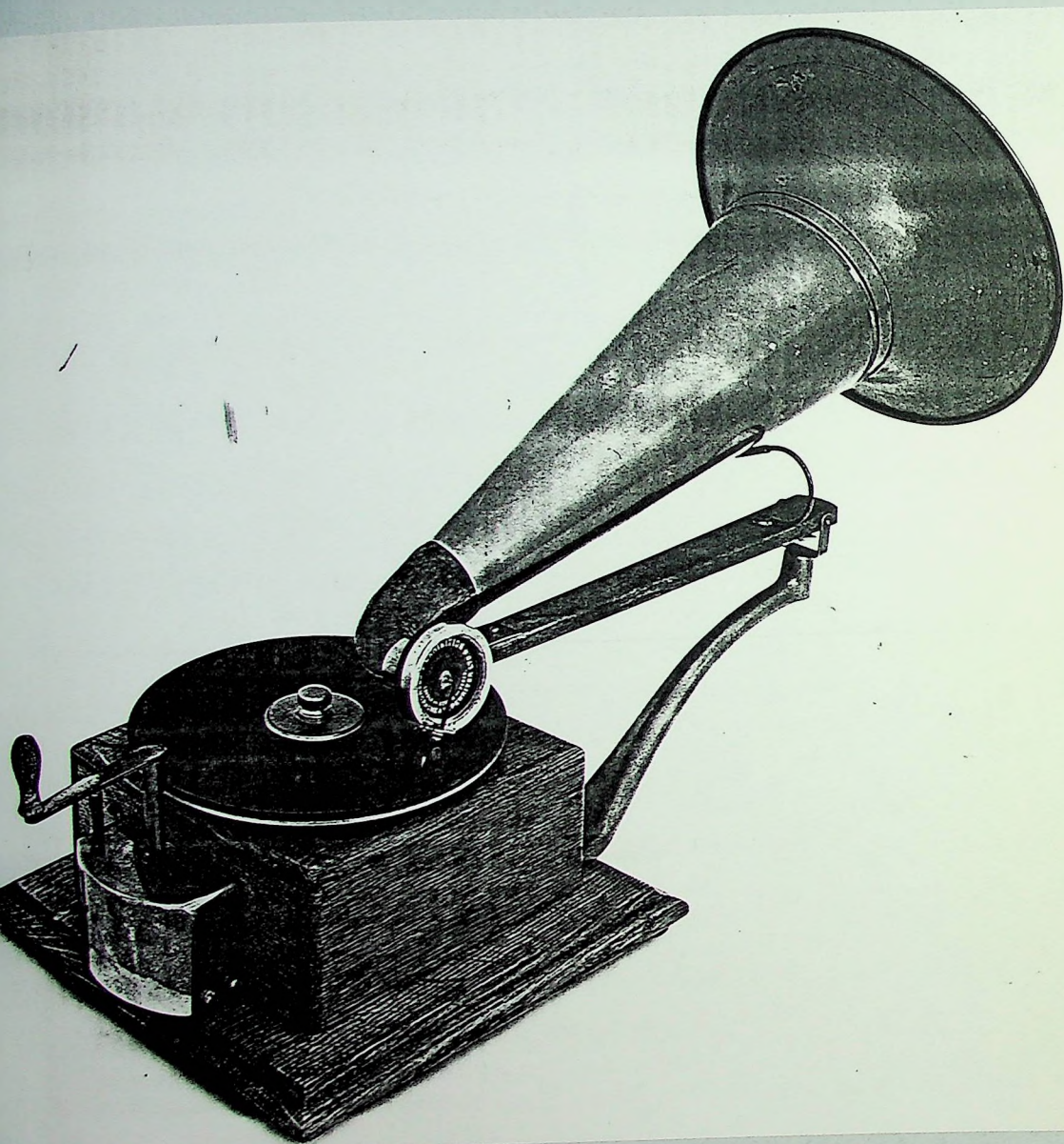
Figure 9: Berliner's first clockwork gramophone sold for $25 in 1895.
