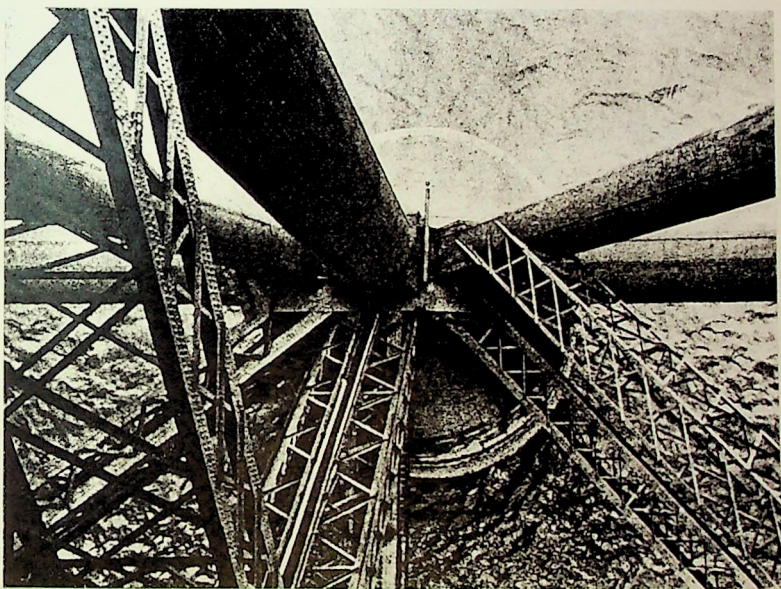
Detail at the foot of one of the main cantilever arms of the Forth Rail Bridge.
