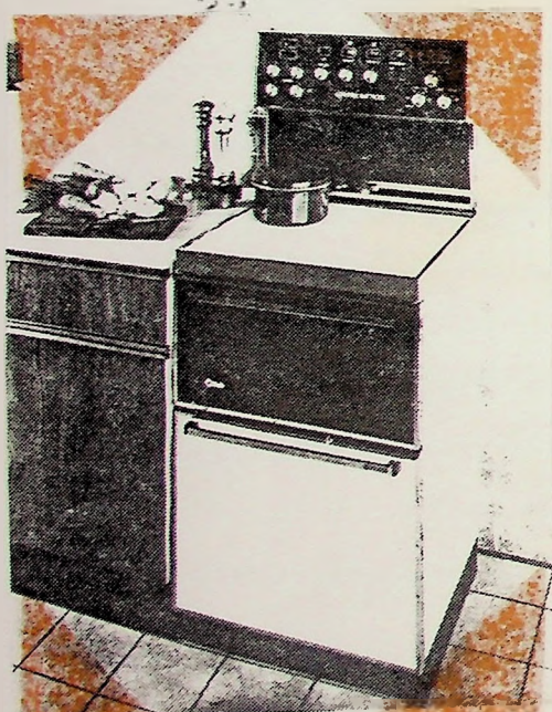
258 Ordo Comfree electronic cooker, 1981. Microprocessor control of cook and timer, six digital display panels, ceramic hob
