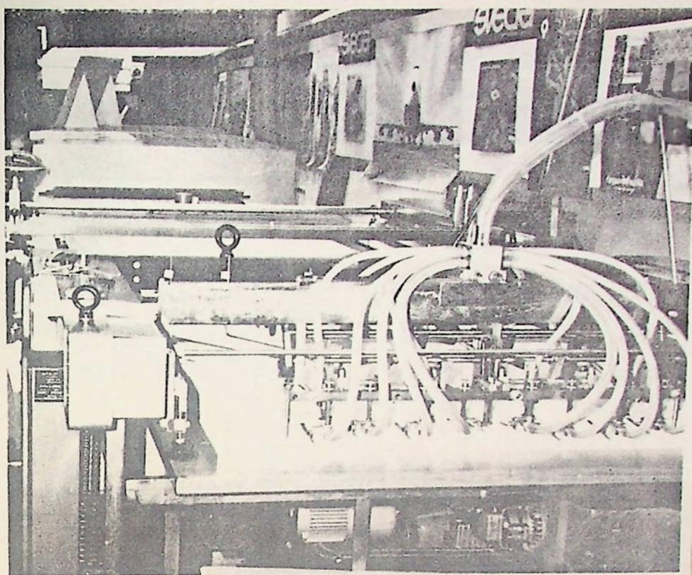
Although conventional printing and drying techniques are likely to be in use for years to come, equipment continues to advance along sophisticated lines. Above is a modern high speed press line with feeder and evaporation dryer.
