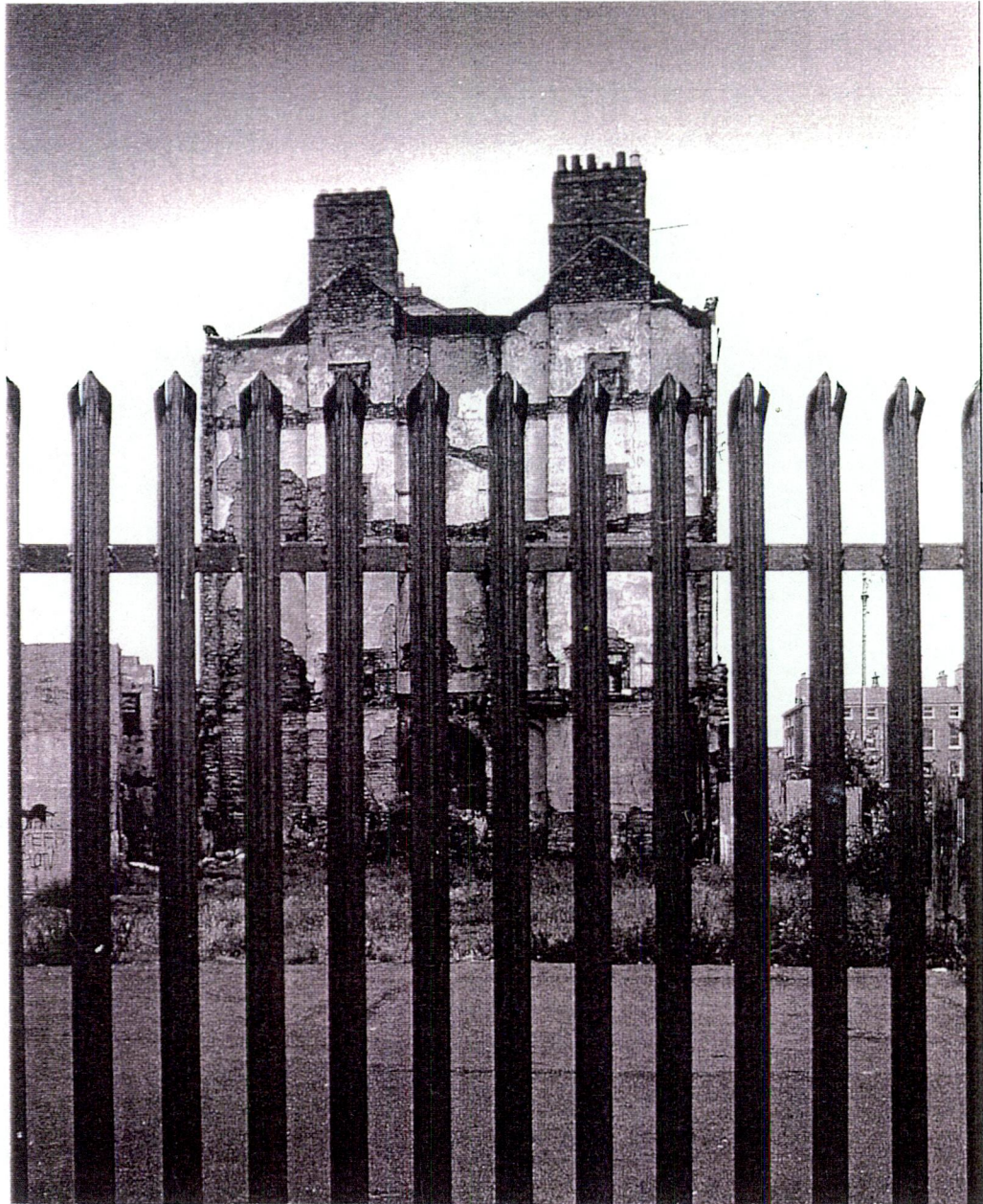
Figure 1.8: What remains of an eighteenth century town house on Mountjoy Square.
