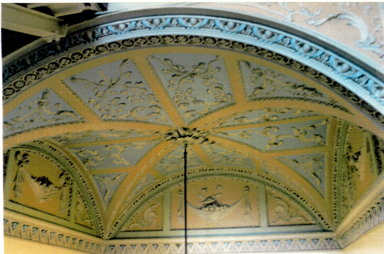
Figure 3.20: The segmented vault ceiling of the outer hallway, no.86 St Stephen's Green.
