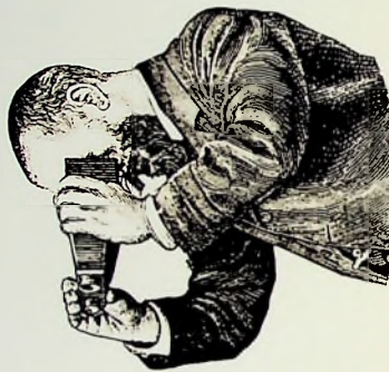
The Photo Jumelle, or Binocular Camera. One lens took the picture while the other lens cast an image for viewing on a ground glass. It held twelve plates 4.5 by 6 cm. Manufactured by Jules Carpentier, Paris. Introduced in 1892.
