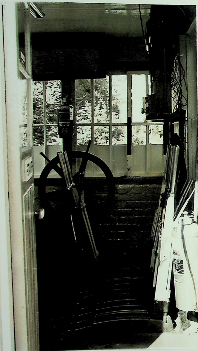
Inside the signal box. Ship-like wheel to open and close gates.
