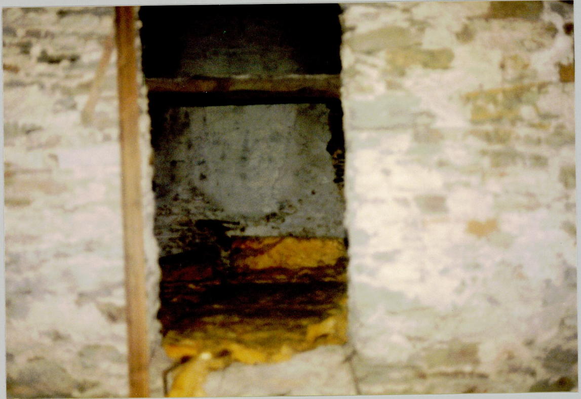
13. Roof-space of main house interior views.
