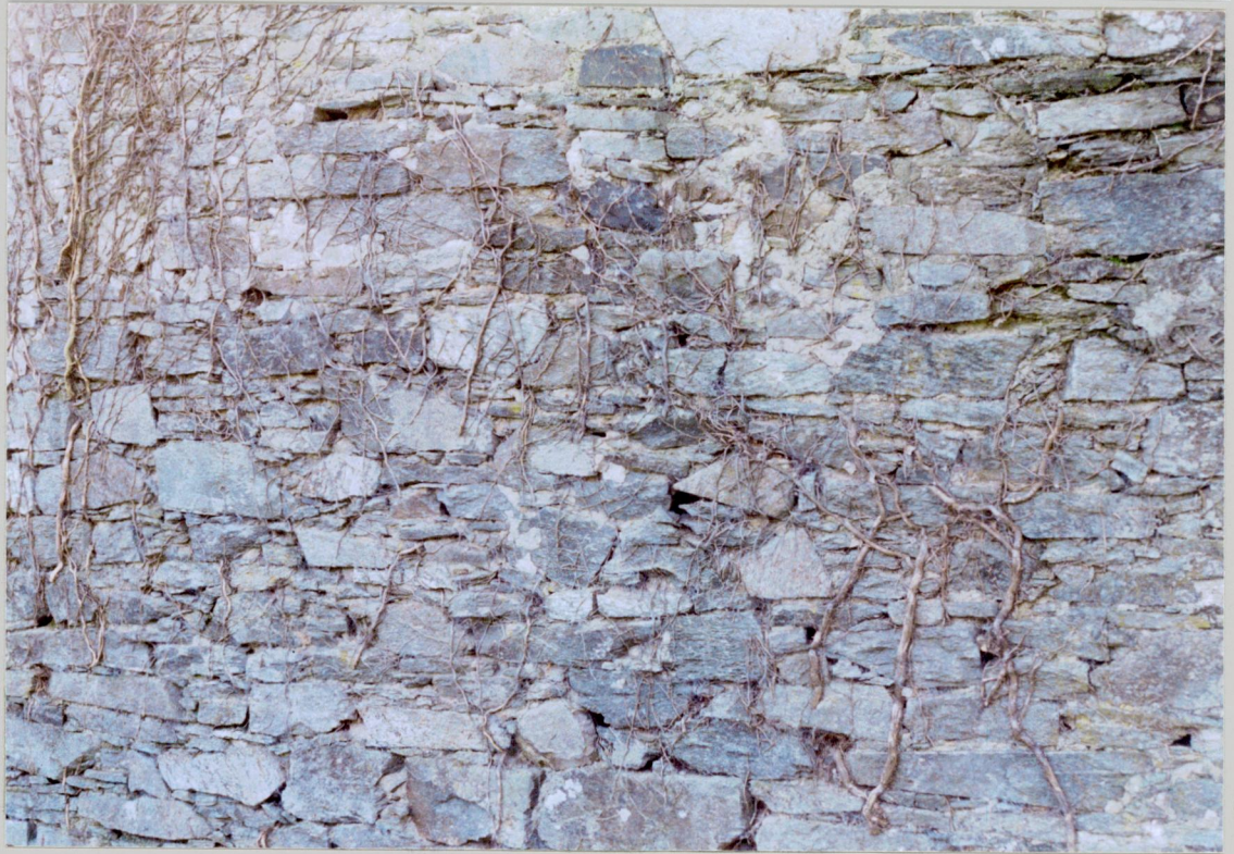
6. Stonework at back of strong-house.
