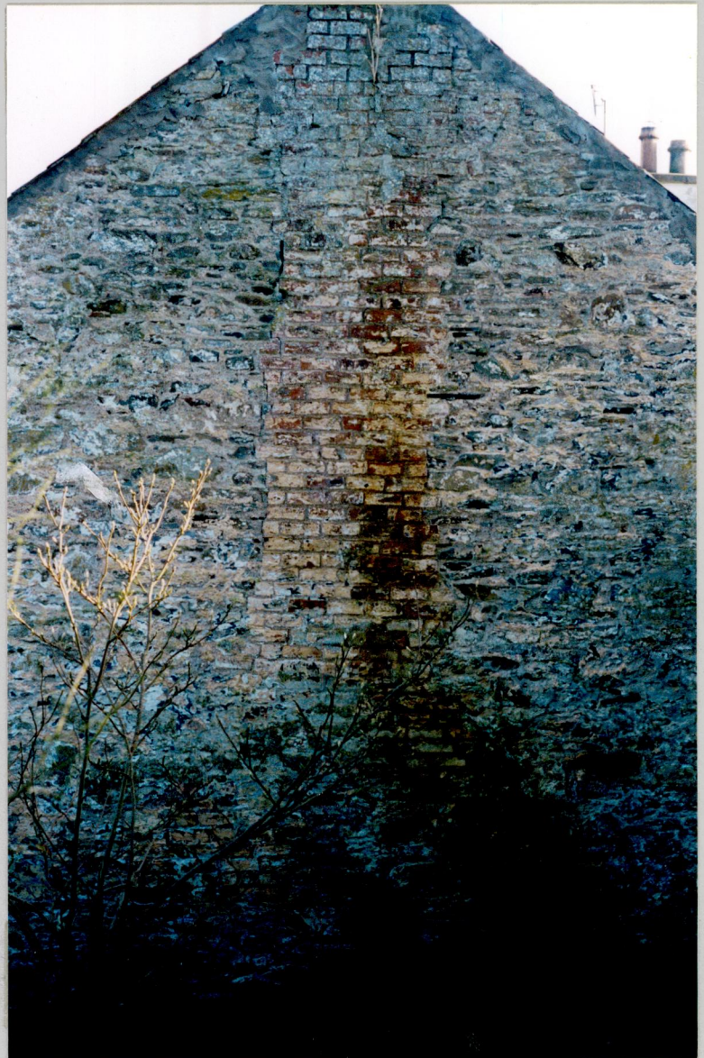
7. Repair work done to chimney breast at back of servant block.
