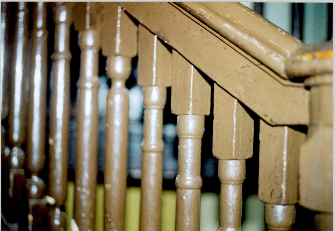
46. Close up view of turned balusters at Cavanacor.
