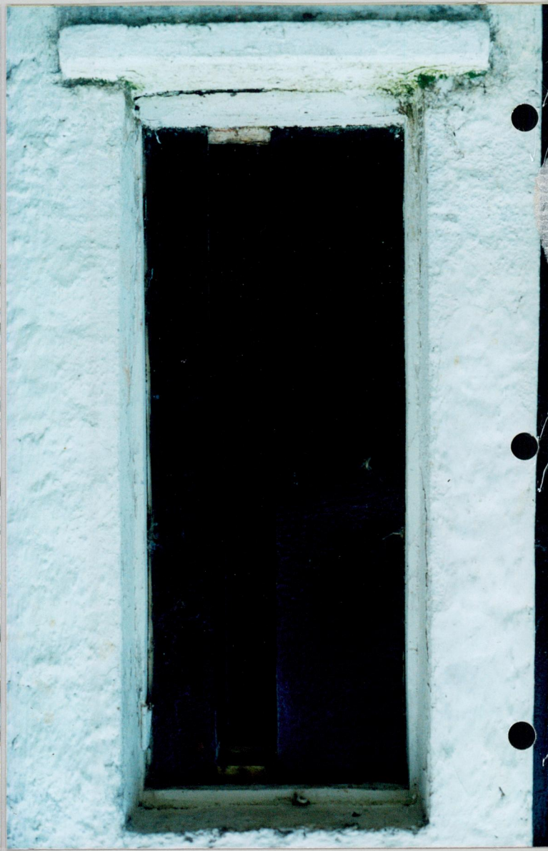
17. Small window in servant block.
