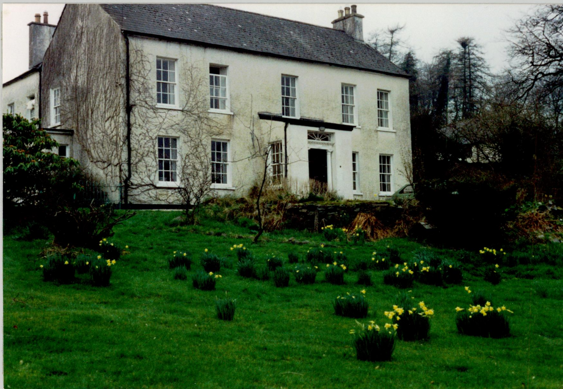
25. Front view of Cavanacor.
