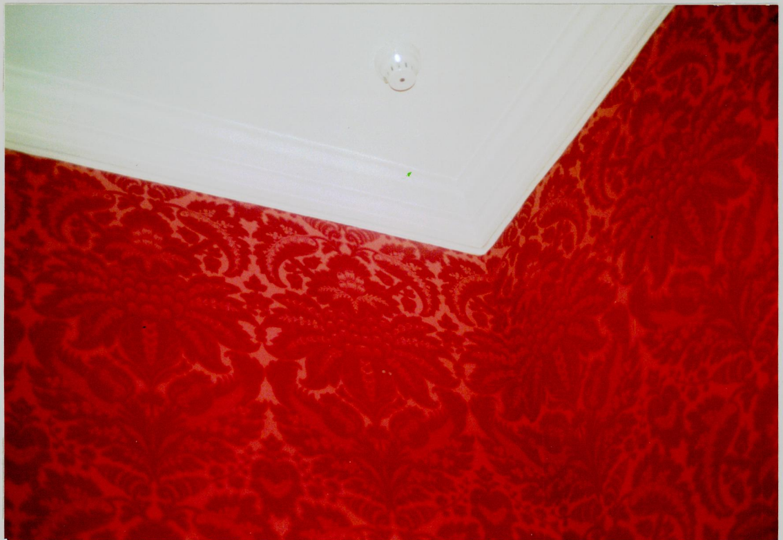
38. Plaster moulding at Springhill.
