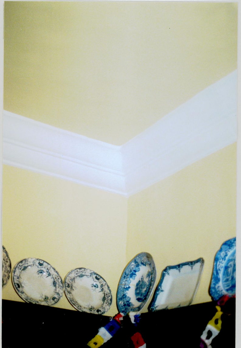
36. Plaster moulding in hall at Cavanacor.
