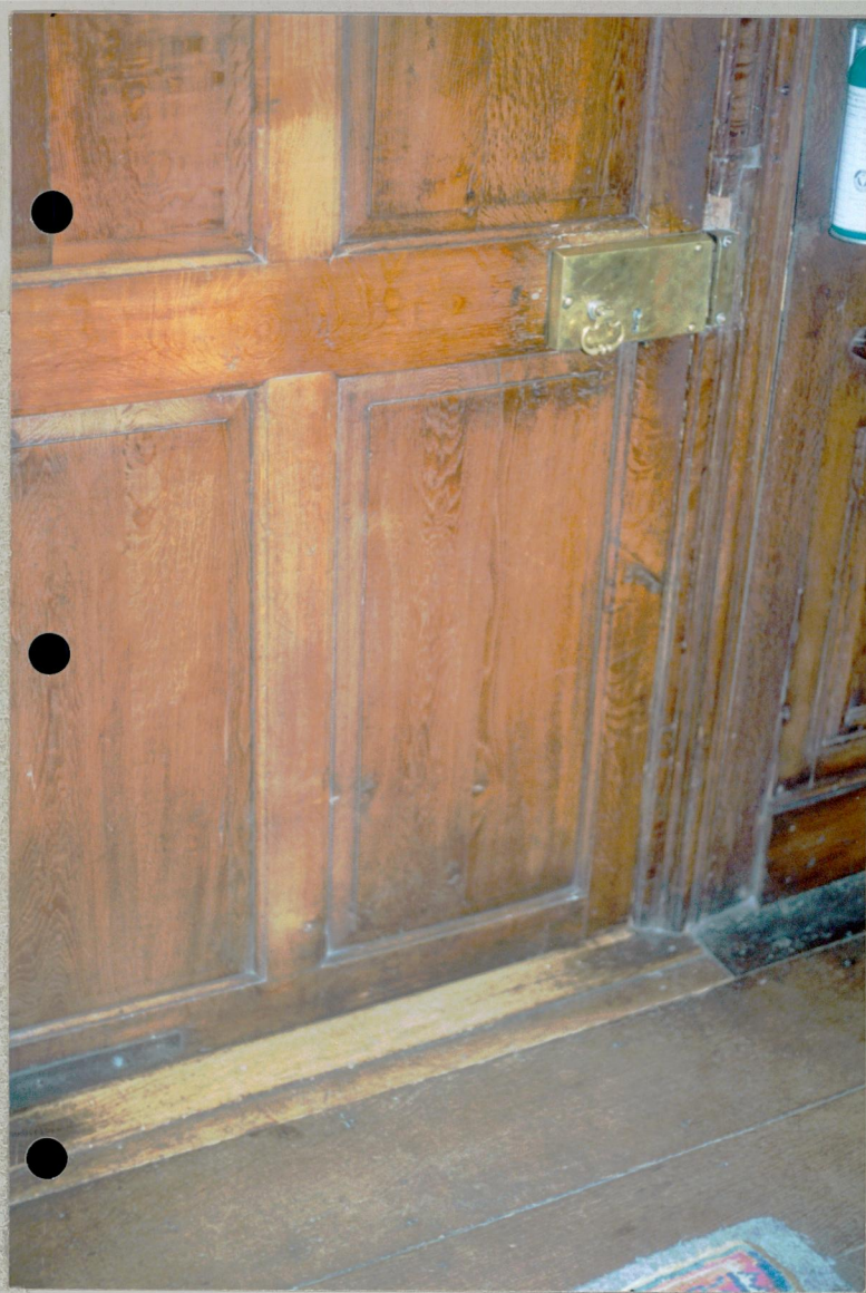
33. Door in front hall at Springhill.
