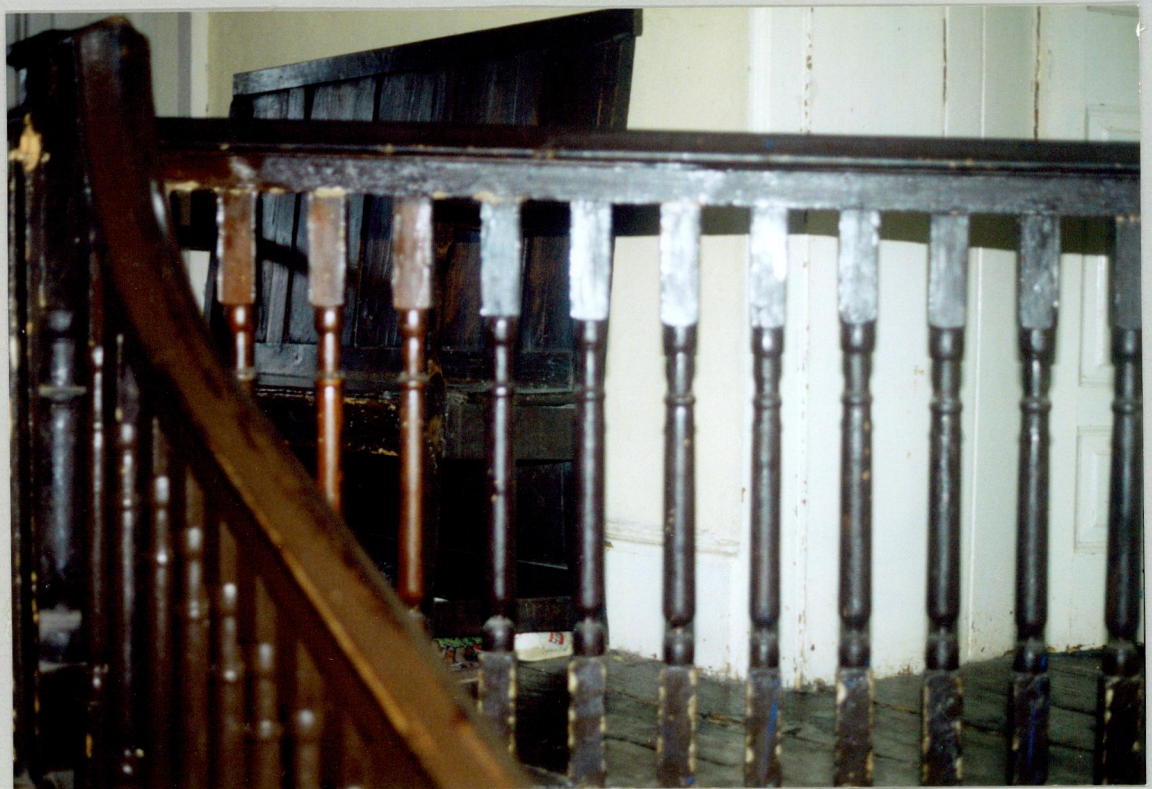
44. Top of staircase at Cavanacor showing part of landing.
