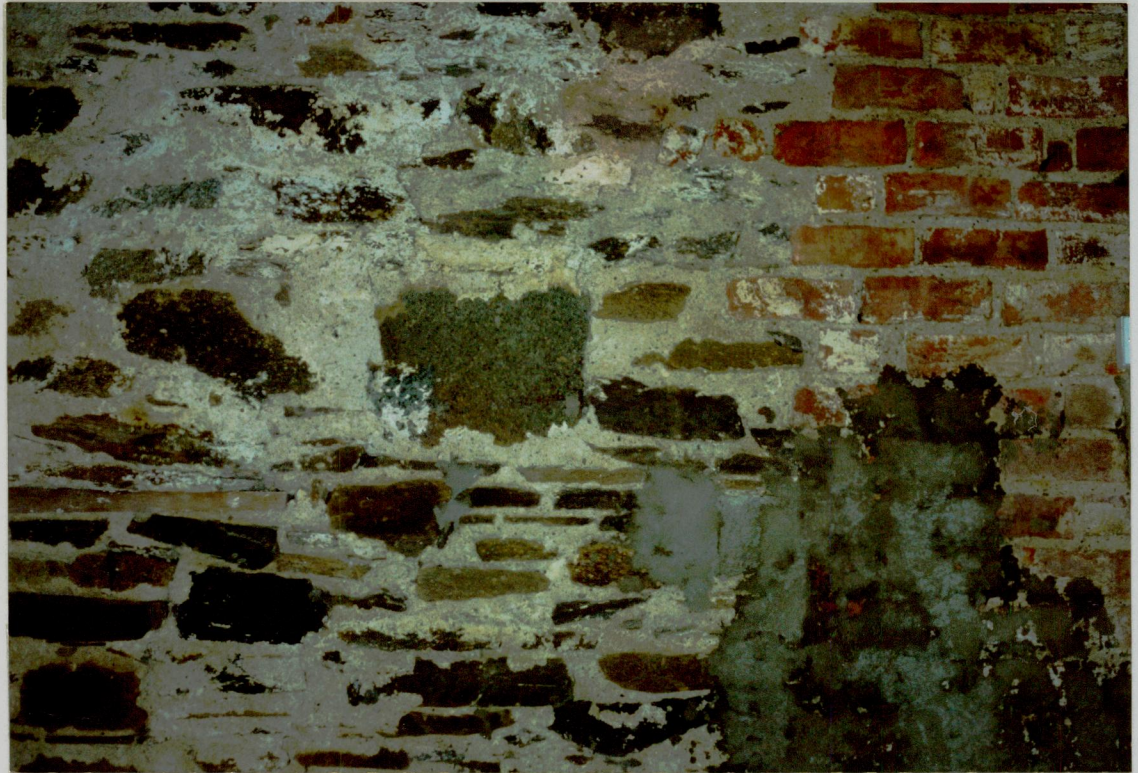
10. Stonework and brickwork in middle wall of strong-house.
