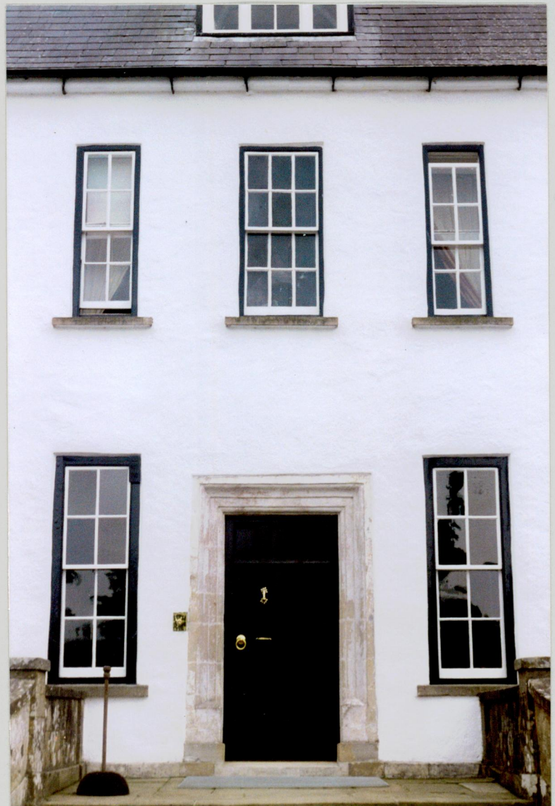
28. View of front door at Springhill.
