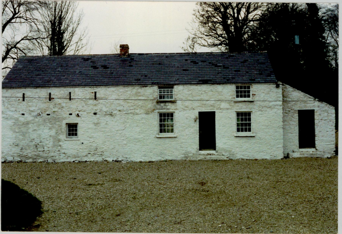
4. Front elevation of building at top of the yard, the strong-house.
