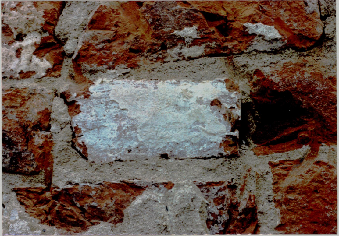
8. Brickwork in middle wall of strong-house.
