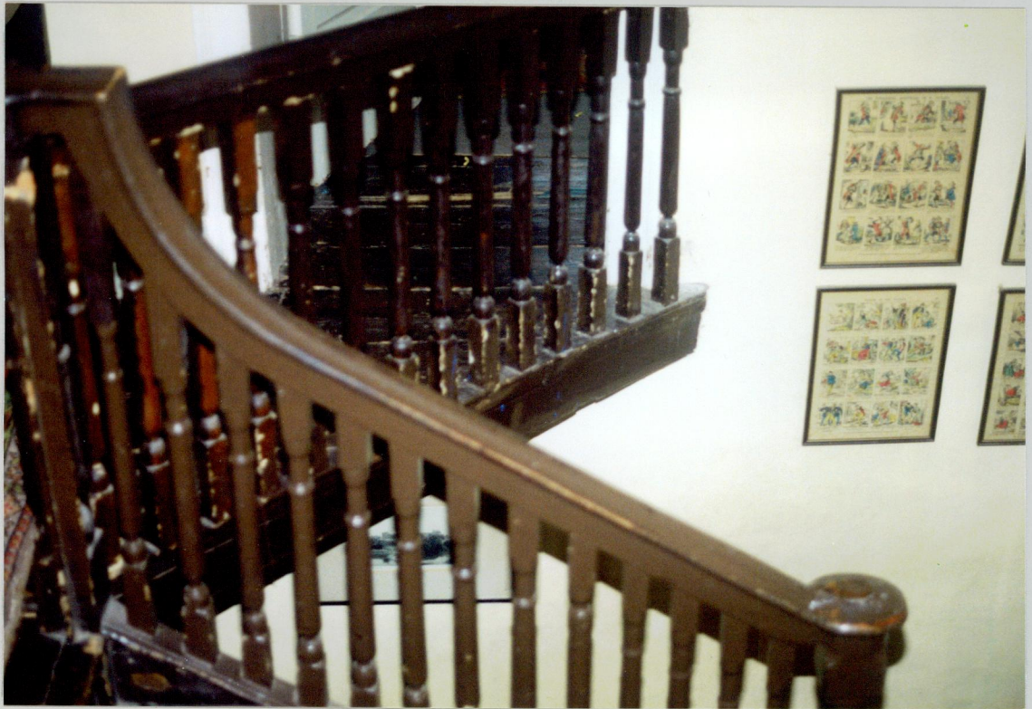
20. Views of 'dog -leg' stairway and cupboard on half landing.
