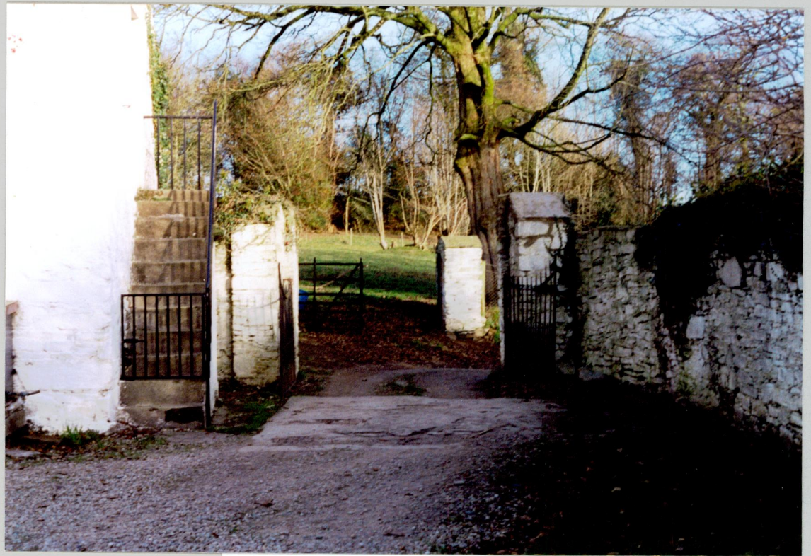
47. View of main gate to yard from yard.
