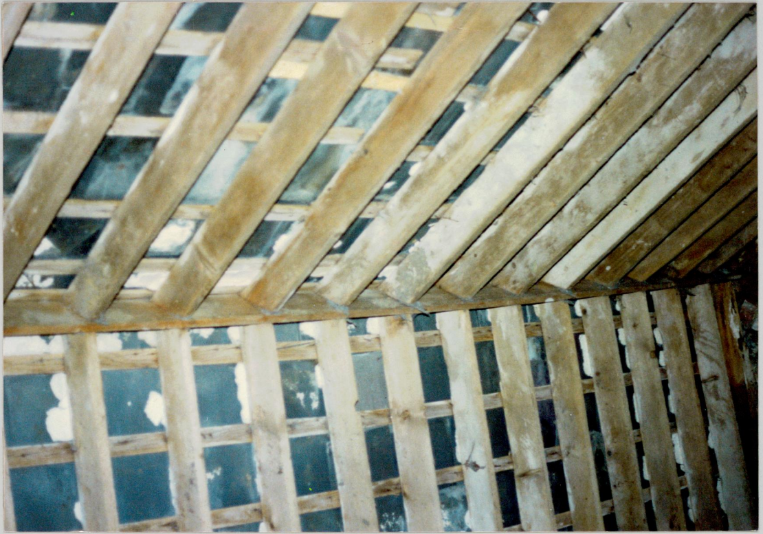
11. Roof rafters in strong-house.
