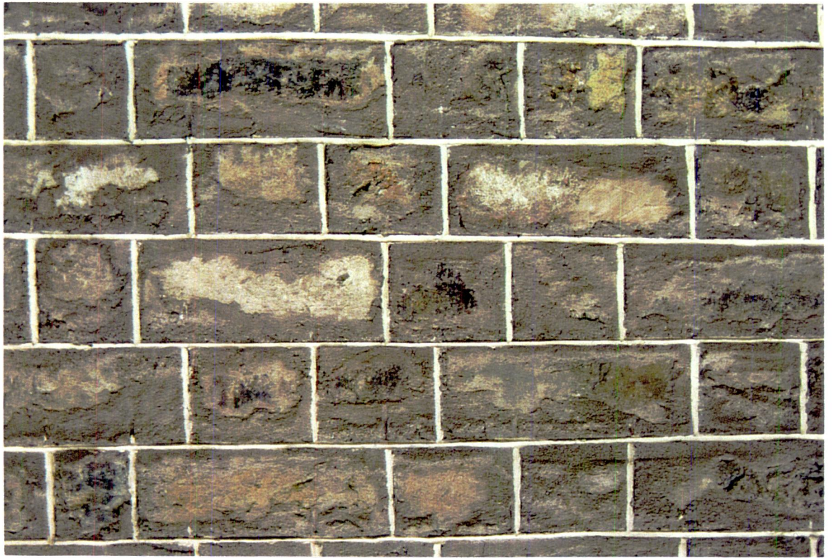
Plate 6. The "pointed" brickwork.
