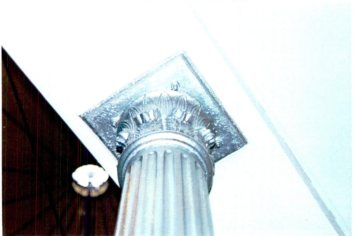
Plate 7. The cast-iron columns.
