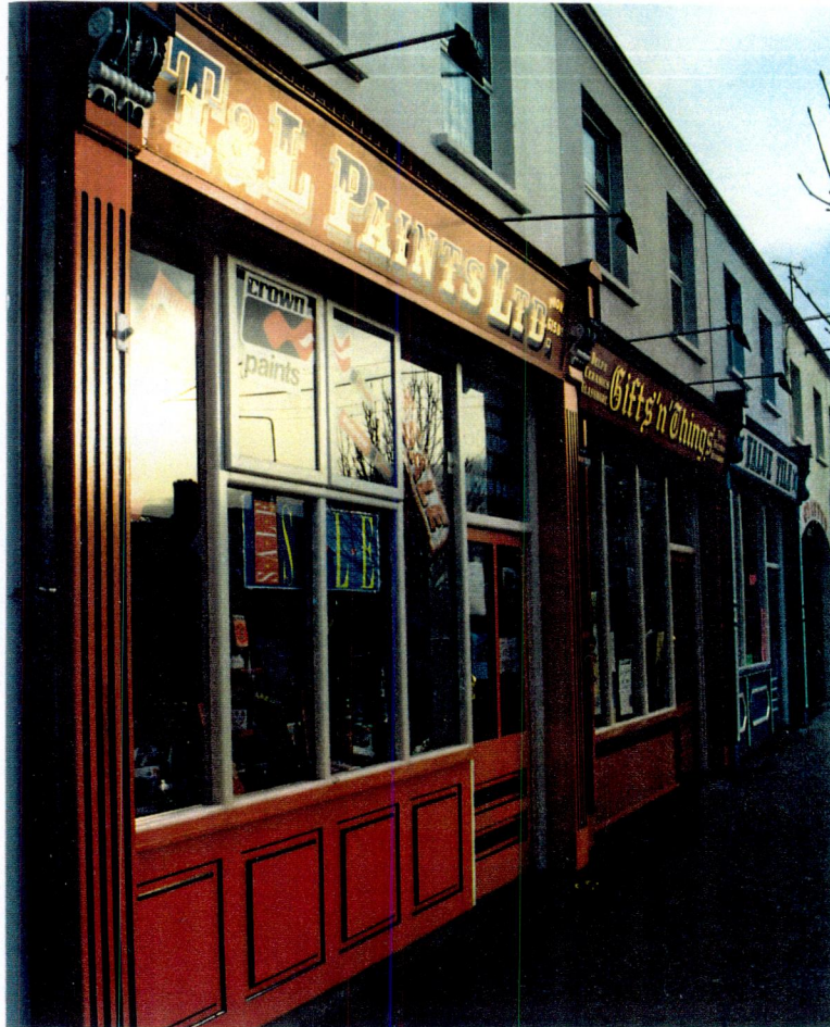
Fig 4.7 A selection of shops on Main Street, Carrickmacross. Spotlights are evident. The shop in the foreground, T & L Paints, was painted by Mr. Larry Martin. The windows are divided into panels by strips of timber.
