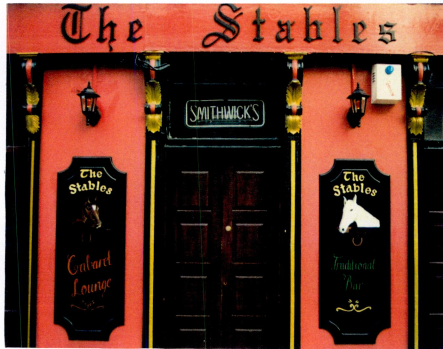
Fig 2.5 The Stables Bar, Main Street, Carrickmacross. The lettering is carved out of wood and painted black, set on a rich salmon pink backdrop. The two panels are hand written.
