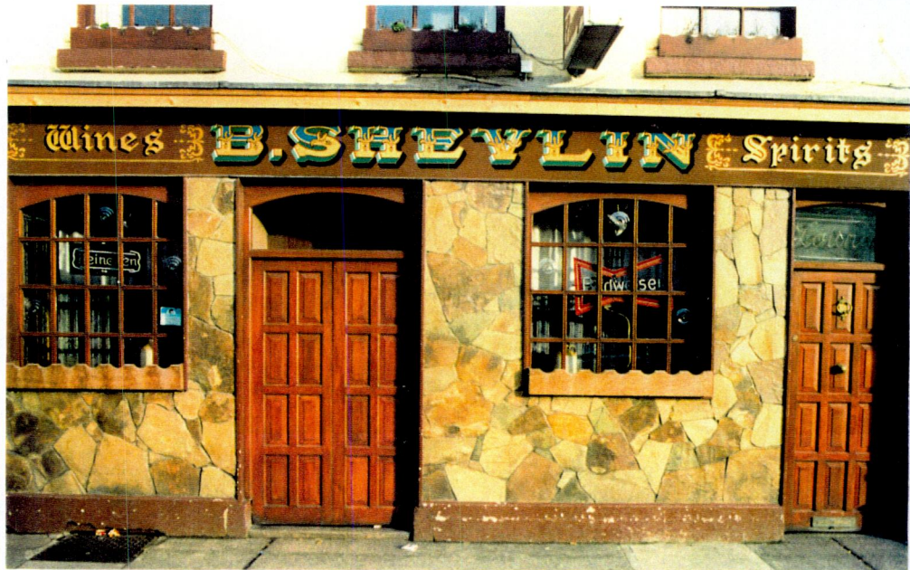
Fig 2.2 Front view of Shevlin's pub, Main Street, Carrickmacross. The natural brown slate is a distinguishing feature.
