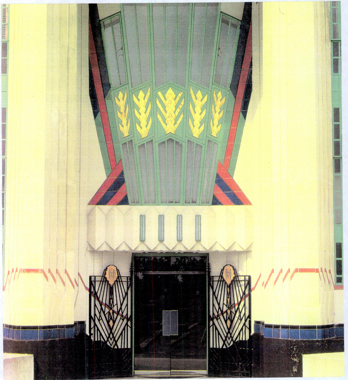
Fig 2. Wallis, Gilbert & Partners, Hoover Building (1932).
